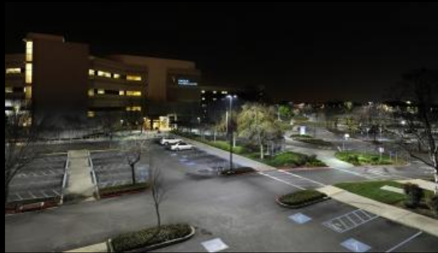
Other area lighting
