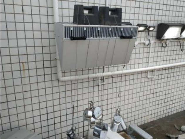
Load bearing Testing
